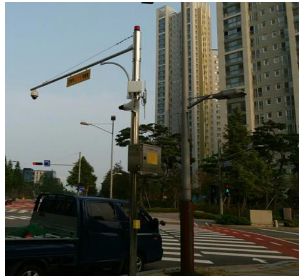
CCTV in Residential areas
