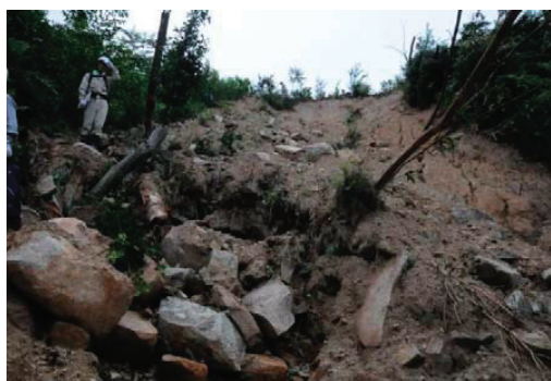
Fig. 1. Source area of a landslide induced by extreme rainfall which caused debris flows which attacked a house for elders in Hofu city.
