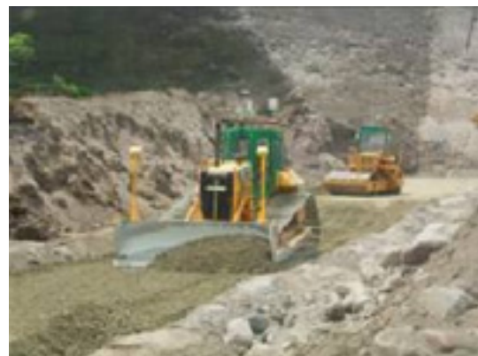
Picture 6 Spreading and compacting of no-slump concrete
