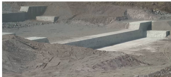
Picture 1 Multilayer sediment control dam
