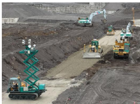
Picture 3 Unmanned construction of multilayer sediment control dam
