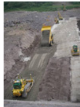
Picture 5 Dumping spot of no-slump concrete
