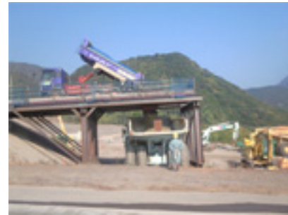
Picture 4 Transfer spot of no-slump concrete
