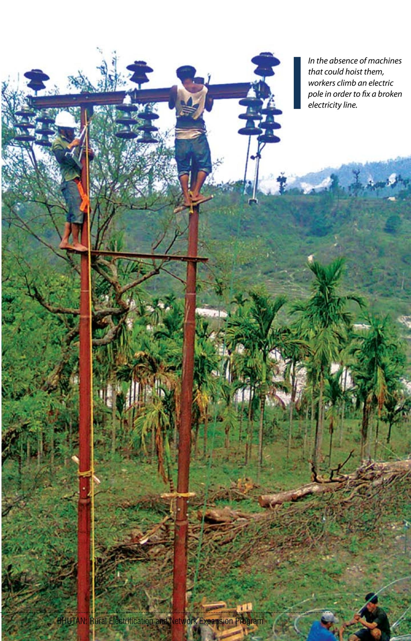
*In the absence of machines that could hoist them, workers climb an electric pole in order to fix a broken electricity line.*
