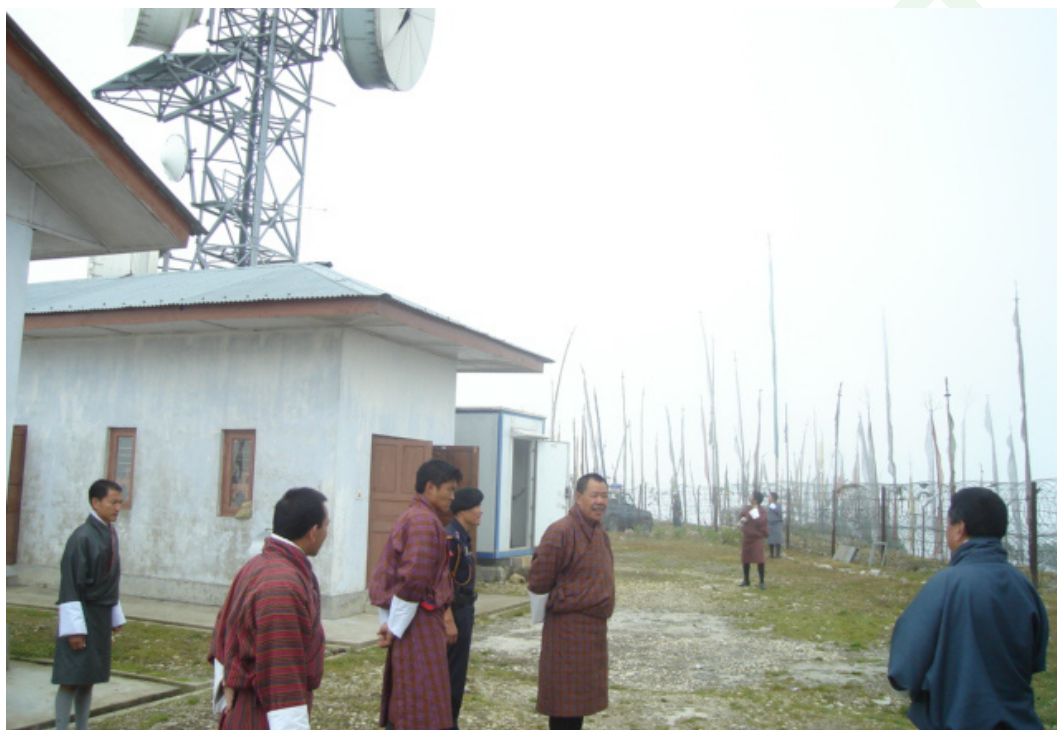
Yongla Goenpa Repeater Station
