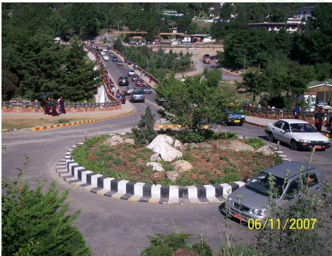
Traffic Flow on the Lungtenzampa Bridge, Thimphu
